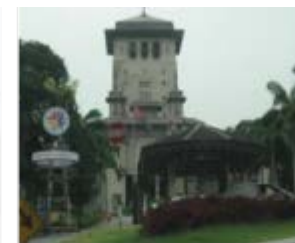
Sultan Ibrahim Building
